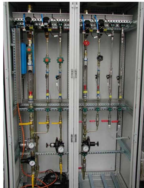
Picture 2: left side = gassing table, right side = gassing cabinet
